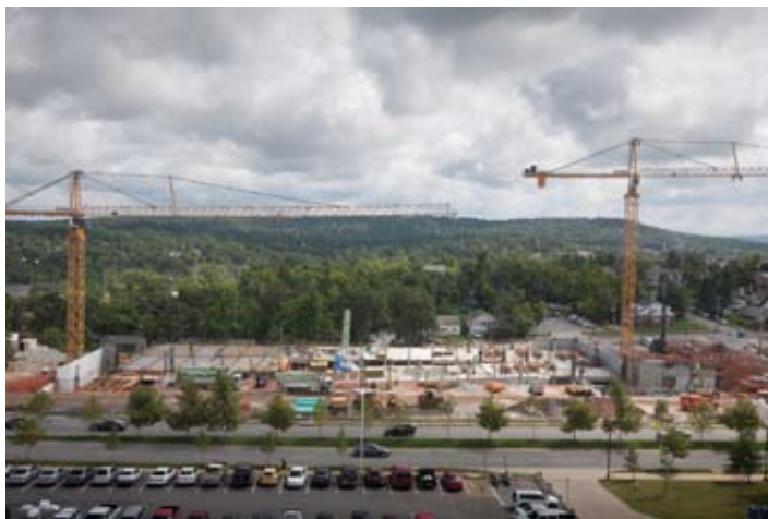
At the University of Arkansas, Fayetteville, twin cranes bring construction materials during erection of the Garland Center, a parking facility along Garland Avenue with retail space for the bookstore.
