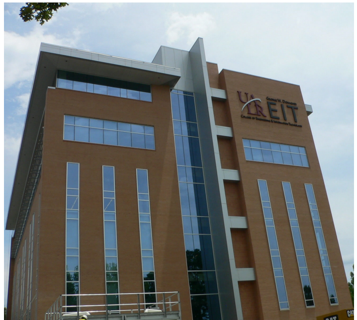
The University of Arkansas at Little Rock's new six-story Donaghey College of Engineering and Information Technology building got under way in 2009, a high performance learning center with an environmentally-friendly focus.
